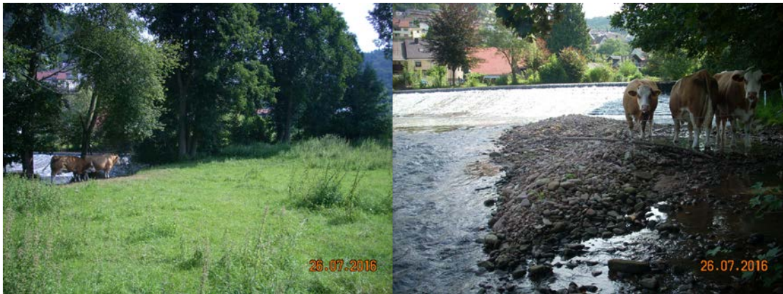
Wehranlage in Eichenbühl
